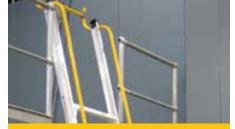
A Safety Gate is provided at the upper floor level to maintain the integrity of the perimeter railing.
